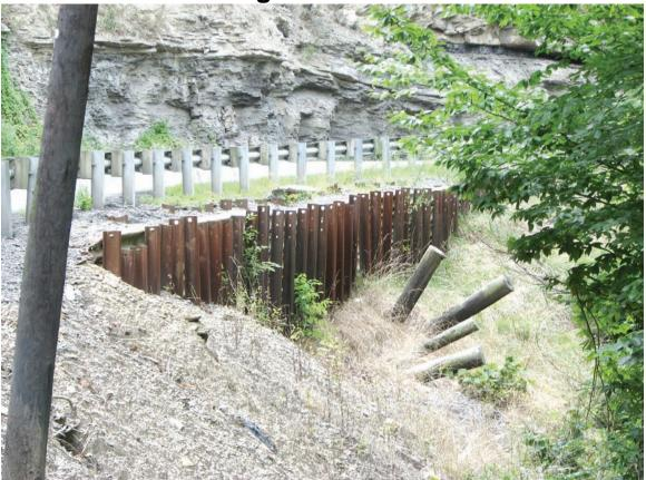
Shales in the Pikeville Formation, exposed here along Ky. 172 in Johnson County, provide a poor foundation and are unstable on slopes; additional support was required to prevent pavement failure. Photo by Dan Carey, Kentucky Geological Survey.
